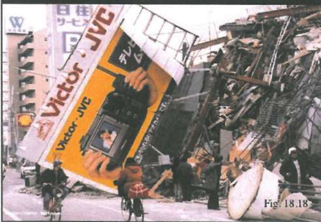
Effects of the 1995 Kobe, Japan, Earthquake
